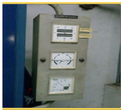
Synchronoscope de couplage
