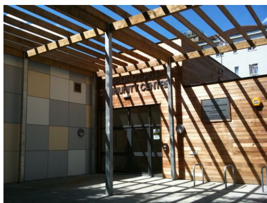
Photographie 12: Tarling East Community Centre
