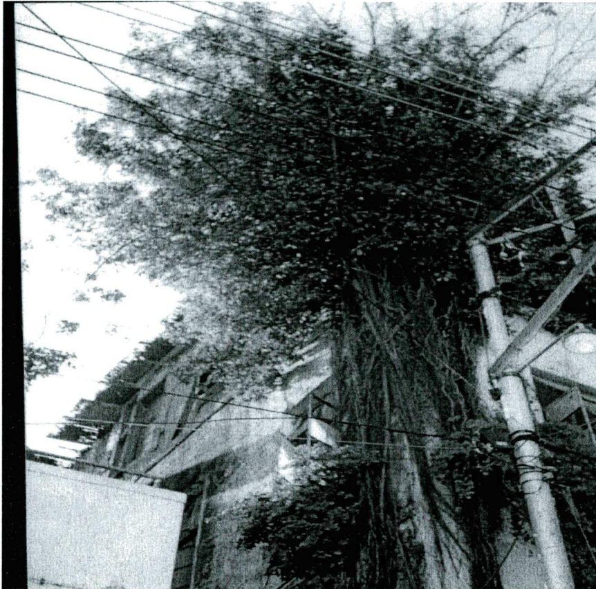
Plate 6.10: Tree Growing On the Wall in the Old town just opposite Fort Jesus.(Source NMK, 2010)
