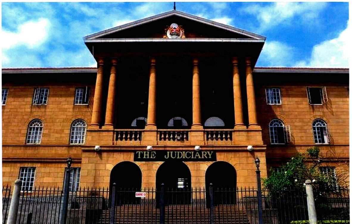
The High Court was built in 1932 to 1934.
