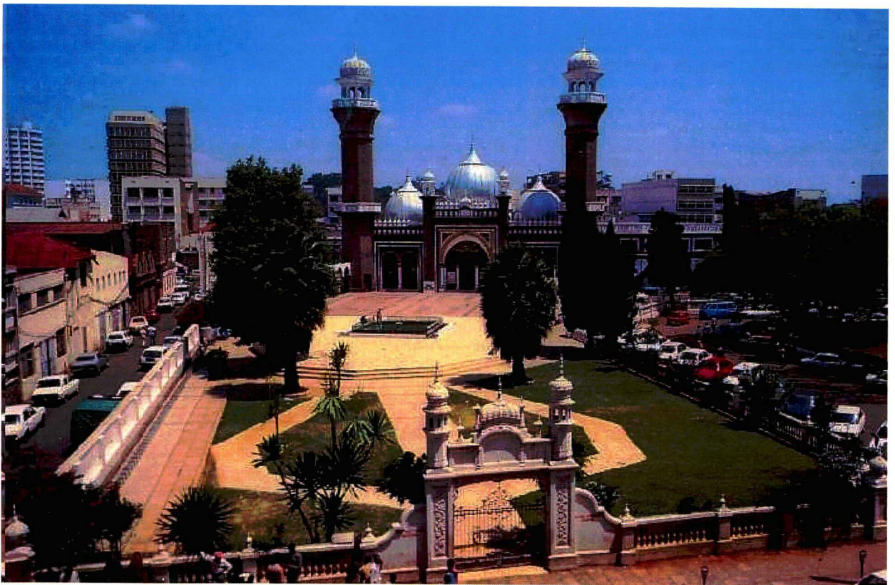
Before the new gateway was constructed
