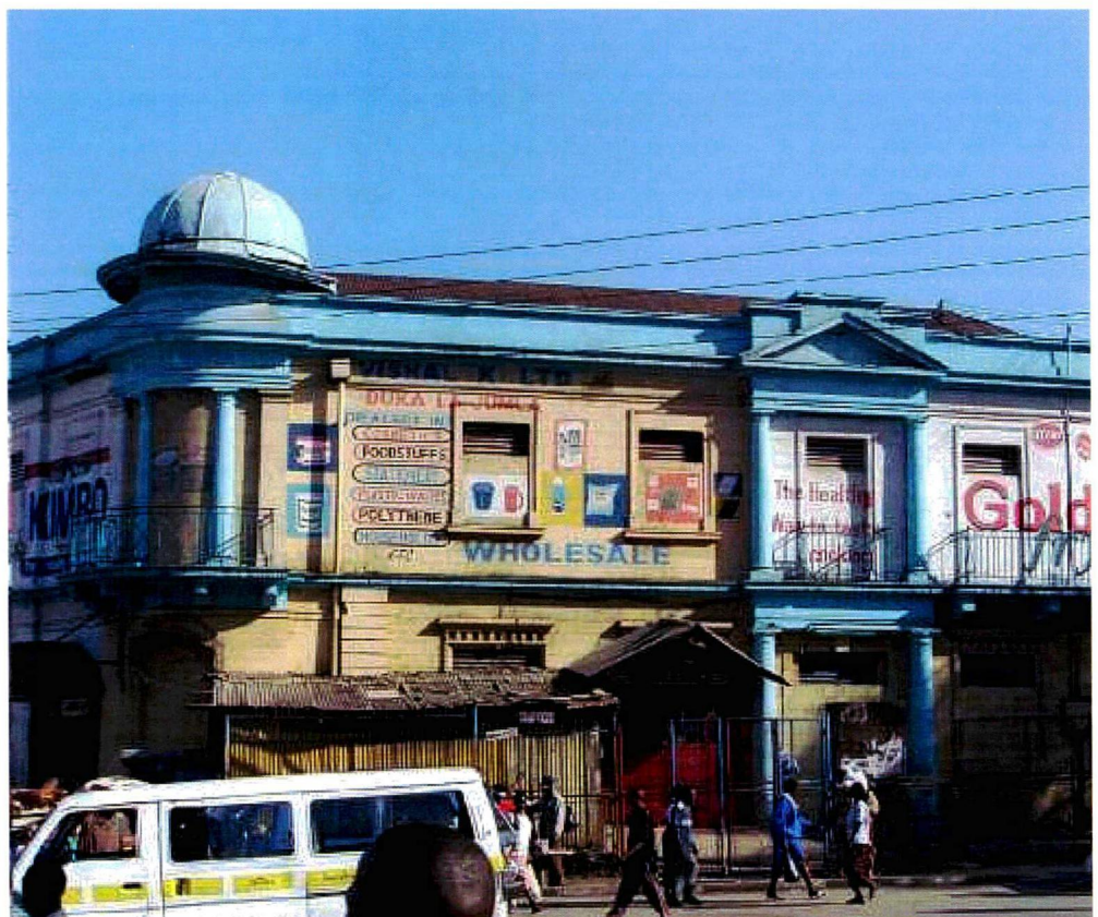
Shop building along Duke Street (today's Ronald Ngala). Built in 1918 according to the date inscribed on the façade.
