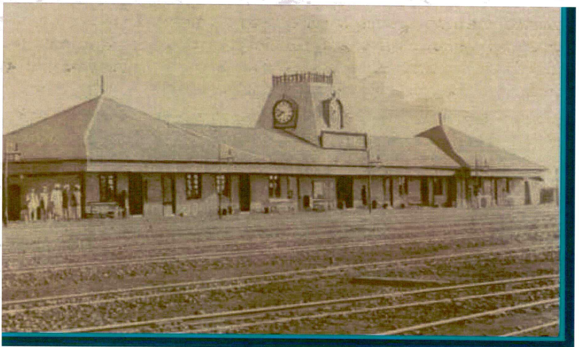
Nairobi Railway Station in 1906. The building is made out of mabati (corrugated iron sheets) and wood. It has since been demolished.
