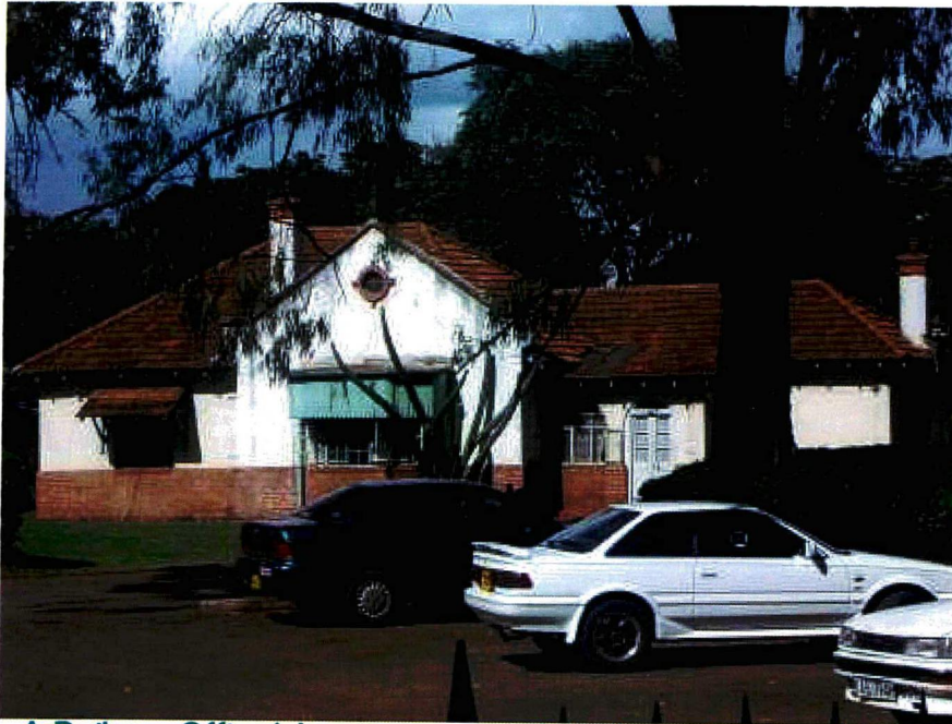
A Railway Officer's house constructed in the early years (1900s) and still standing
