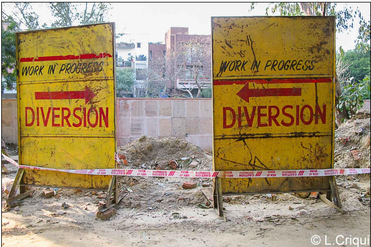
Photo 1/D. Work in progress (Delhi, 09/02/2013)
