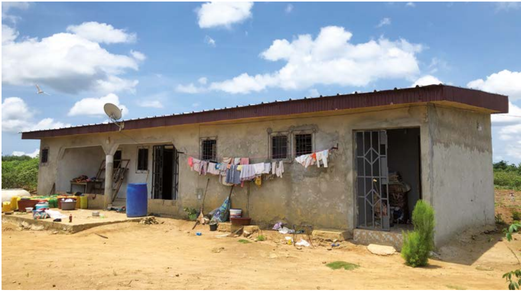
Construction on newly parcelled land in Djimini-Koffikro, Côte d'Ivoire, 2023 © Colin
