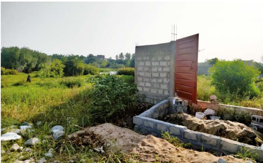
Fenced subdivided plot on the edge of the lagoon in Togbin, Benin, 2021 © Simonneau
