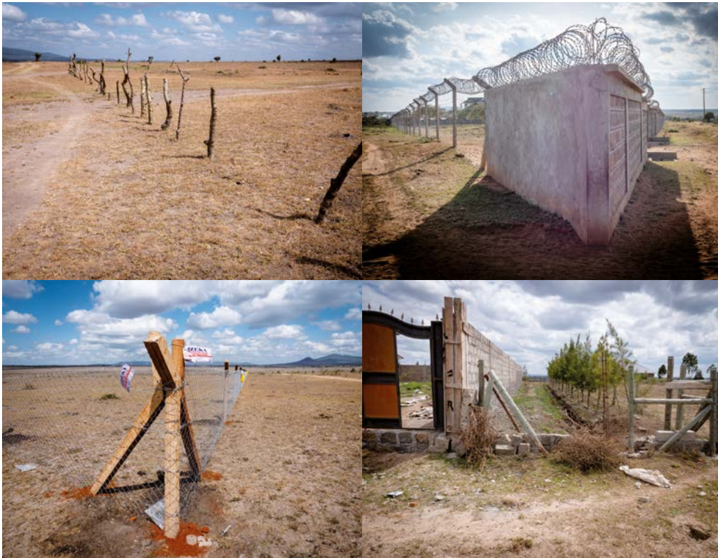
Examples of markers and fences in Kenya: bits of wood, posts, barbed wire, walls, line of trees and gate, 2022 © Bon
