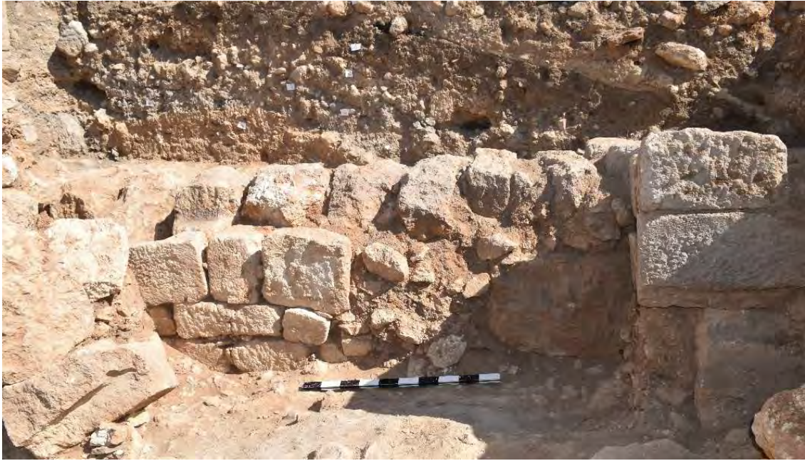
Fig. II.16. Northern wall (W60) of room R1.
