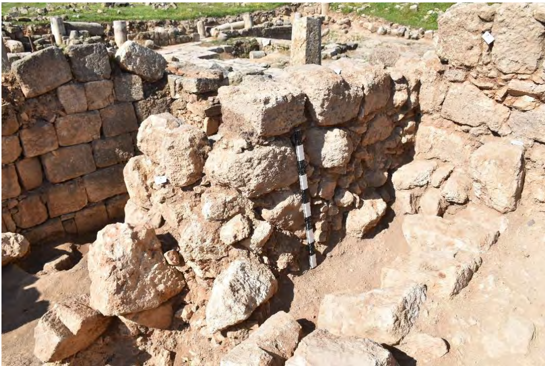
Fig. II.8: Corner between walls W45 to the right and W66 to the left, view from the northeast.
