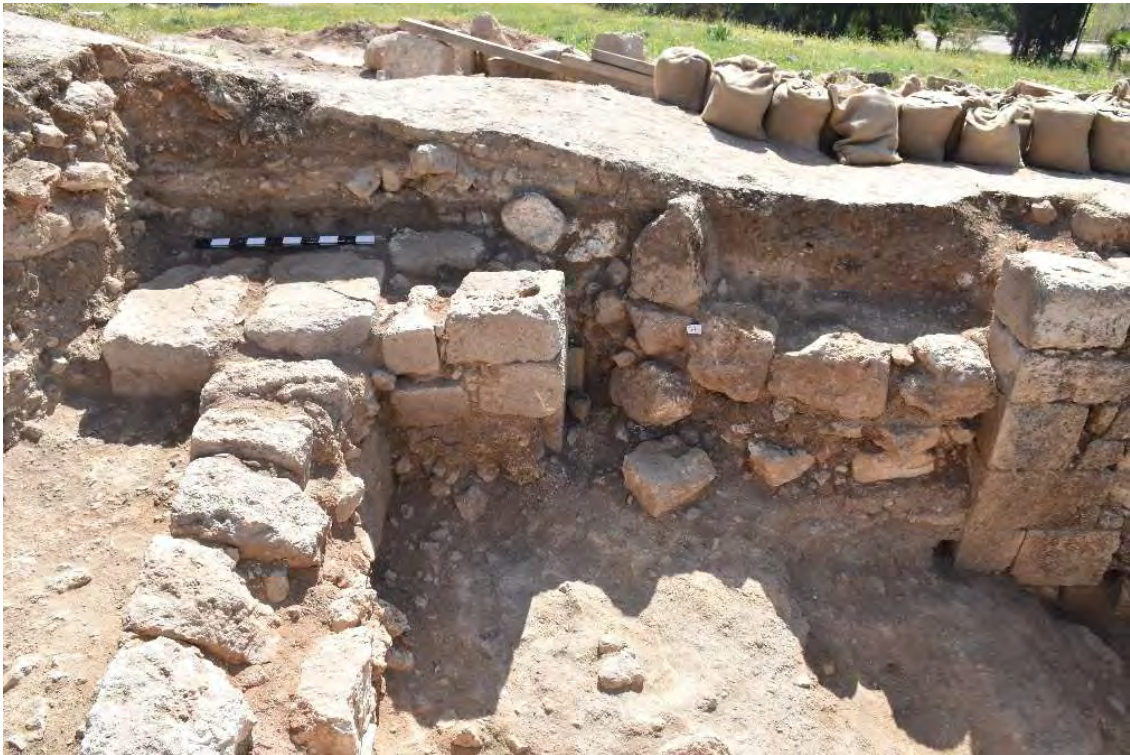
Fig. II.19: Wall W1 continuing to the north and door of building A. W65 that was later added to condemn the passage.
