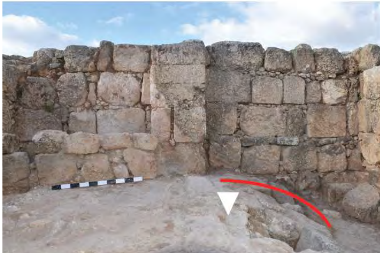
Fig. VII.19. Support by retaining vault (room R4).
