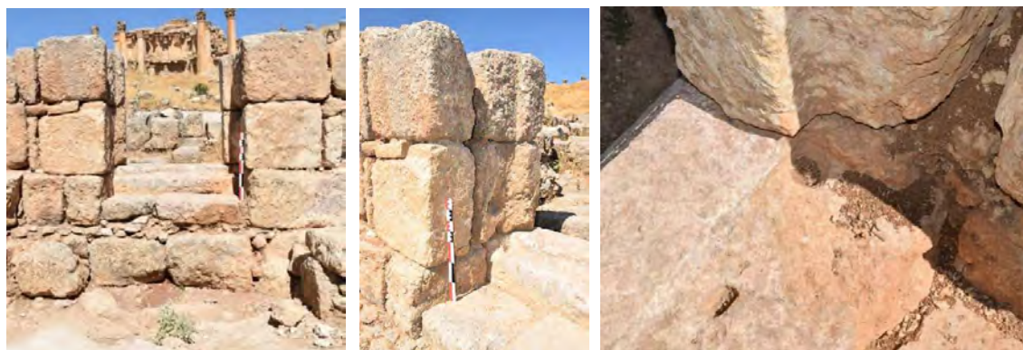
Fig. VII.15. To the left, elevation of the access bay in room R4; in the middle, the door rabbet in room R4; to the right, door sockets.
