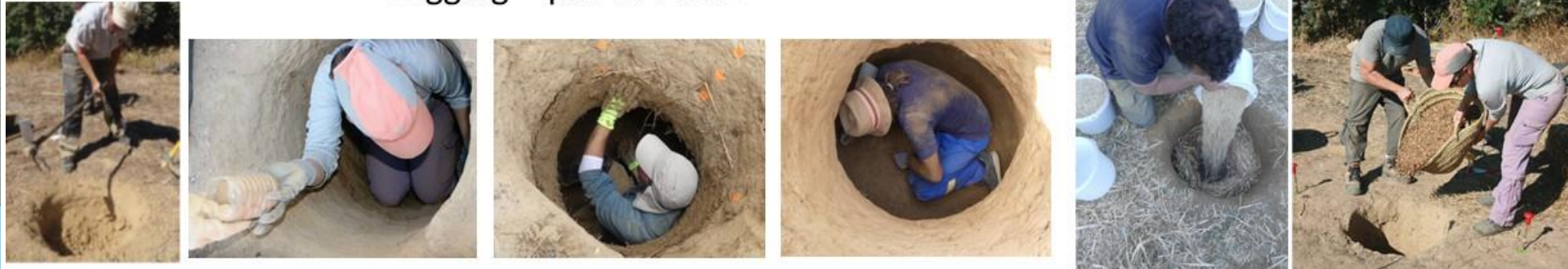
Digging – pits of 700 L
