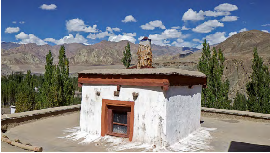
FIGURE 12 The Tsa Tsa Puri temple, located in Alchi next to the Indus River, probably dates from the fifteenth century. The temple is mostly made from poplar, while the floorboards are made of juniper.
