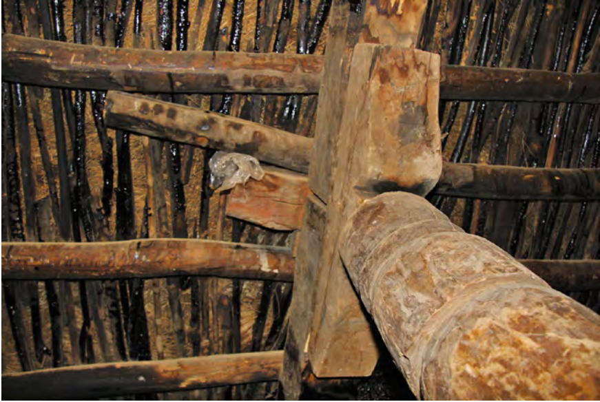
FIGURE 4 Main pillar (poplar wood) and a bracket made of willow. The purlin is made of poplar. The rafters and ceiling-covering sticks (called “ talu ”) are made of willow. The sticks are cut from poles of pollarded willows. Continuous lopping of the top of a tree encourages fresh growth into new shoots producing poles (Corkhill 1979).
