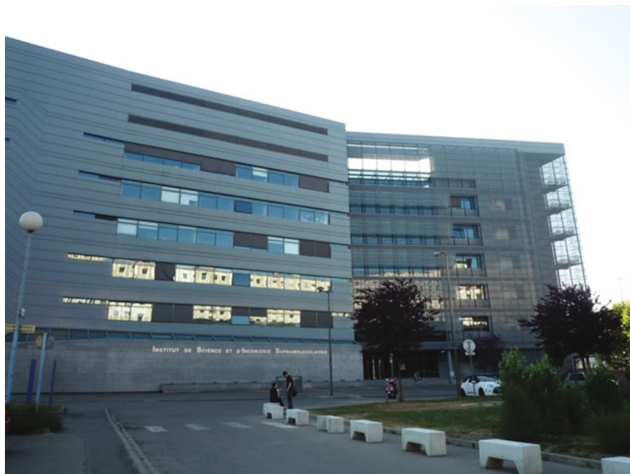
Fig. 2.2 The ISIS building at the University of Strasbourg
