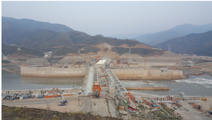
Figure 7: The Xayaburi Dam under construction in February 2018 (Credit: C. Middleton)
