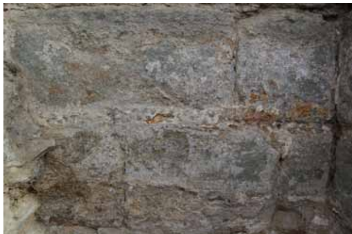
Fig.22: Detail of the overthickness joint with the basalt inclusions (JB 2014).
