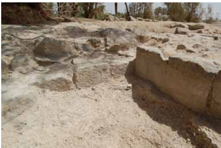
Fig.38: Detail of the connection between walls M3 (in front) and M8 (on the right) in sounding D2 (JB 2014).
