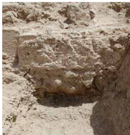
Fig.36: Detail of M3 foundation in sector D (JB 2014).
