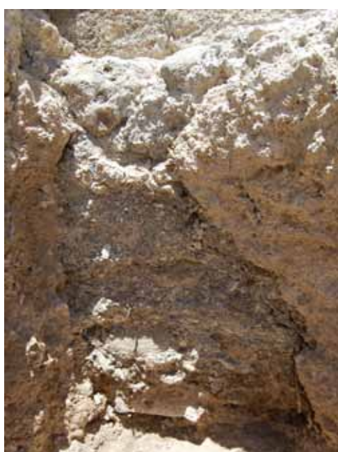
Fig.20: Detail of the foundation in B2 under wall M4 (JB 2014).
