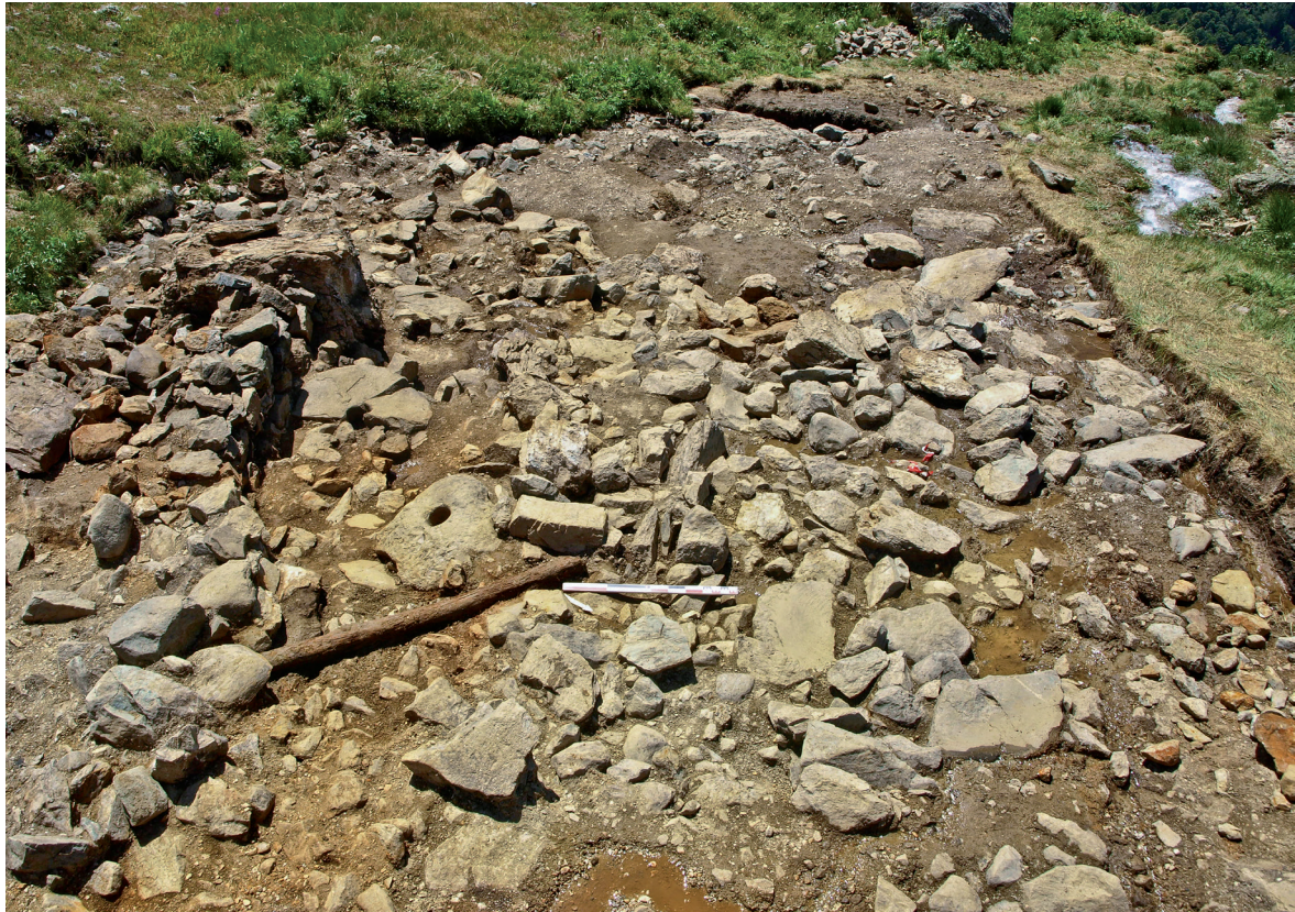
Fig. 3: View from the north-east of the upper layer of demolition of the hydraulic ore mill. A few mill features begin to appear (photograph by N. Minvielle Larousse).
