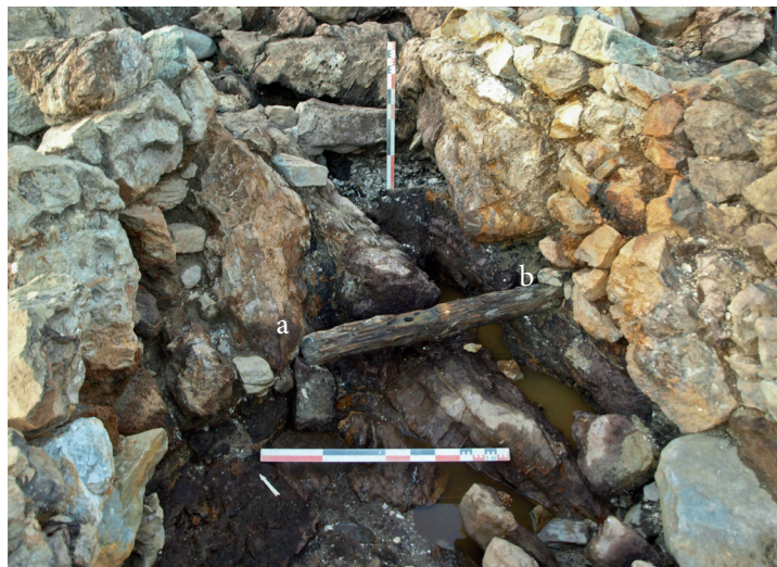
Fig. 17: View of the wooden beam with the central socket separating the flume from the undercroft (photograph by N. Minvielle Larousse).
