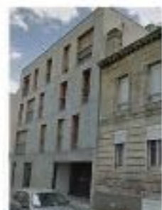
11.17. 118 rue Maube © Google street View
