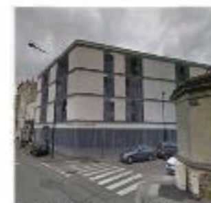
11.19. 112 boulevard Albert 1er © Google street View
