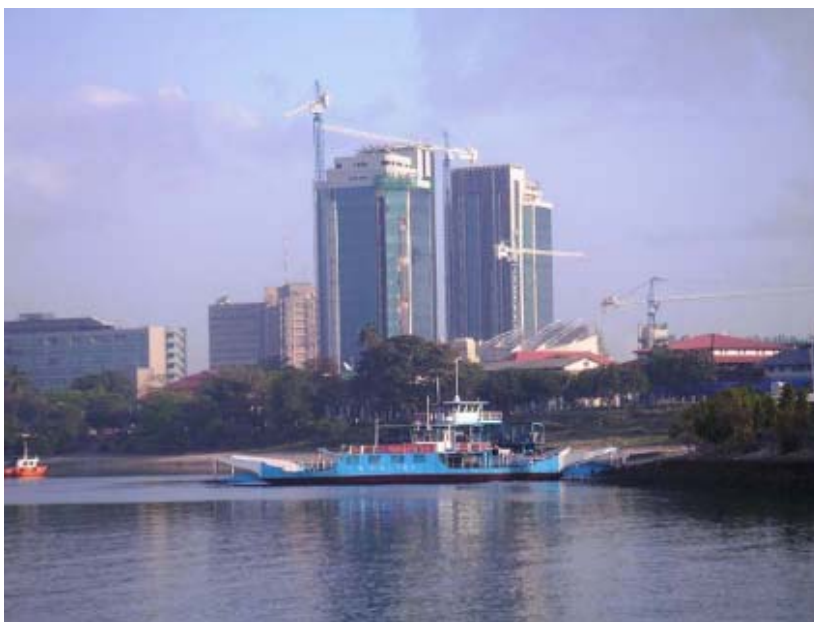
The Central Bank of Tanzania twin towers under construction Dar es Salaam 2005
