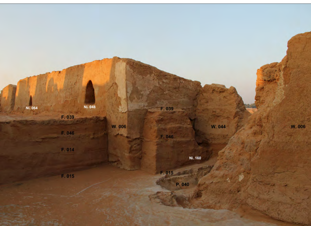
Figure 121 Building 1 – Mihrāb (Ni. 160) in the qibla wall (W. 006), looking southwest (Th. Sagory – French-Saudi Archaeological Mission in al-Kharj)
