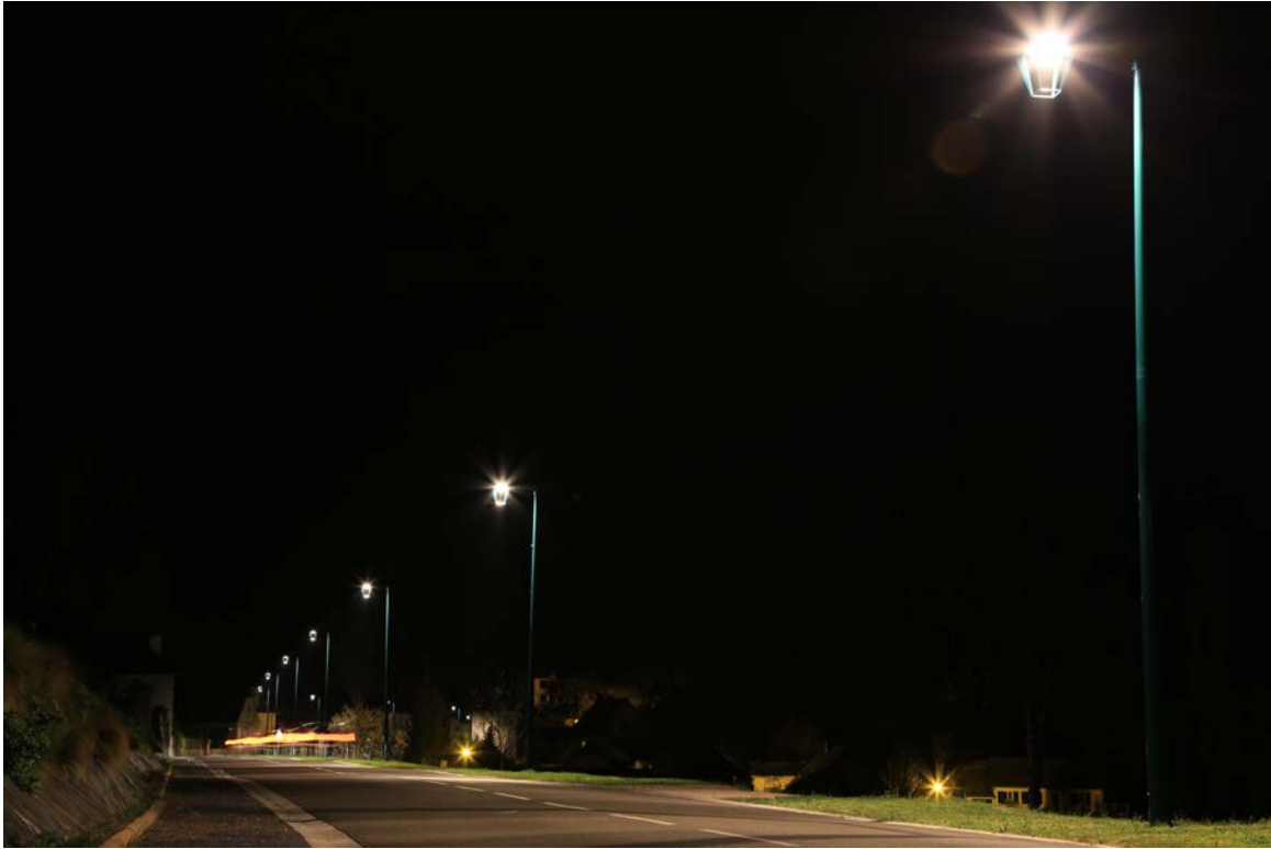
Main street of Agos Vidalos. Full cut off lights, ceramic metal halide lamps with good spectral quality (less proportion of blue), 2800 °K; 10 lux.
