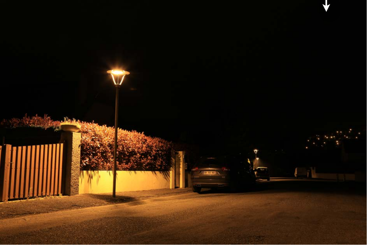
Full cut off lights; hight pressure sodium lamps; 2200 °K; 6 lux.
