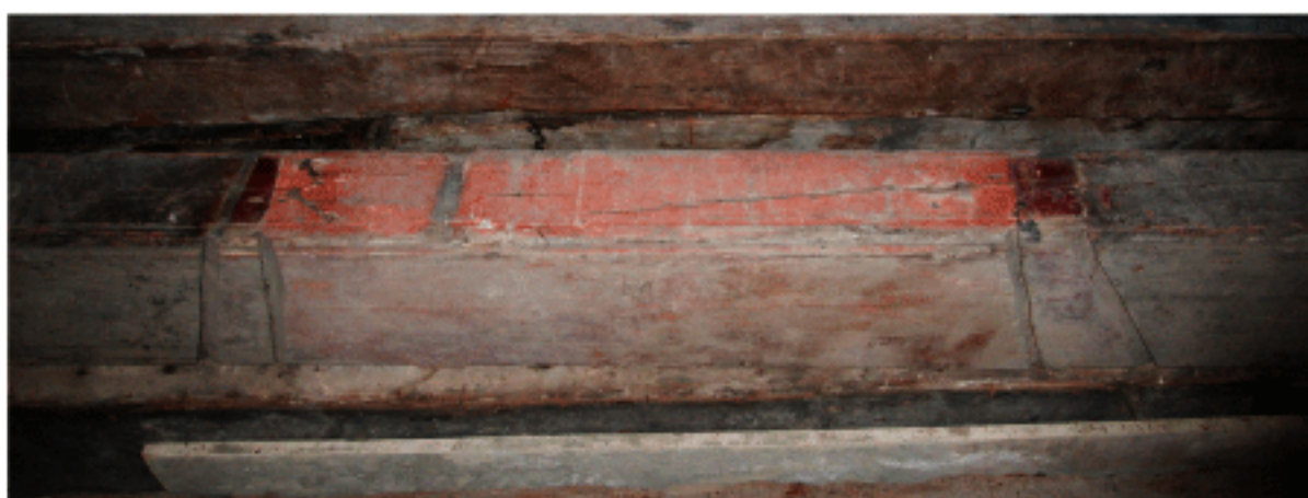
Solive à rainures doubles (cliché P. Maritiaux, LA3M).
