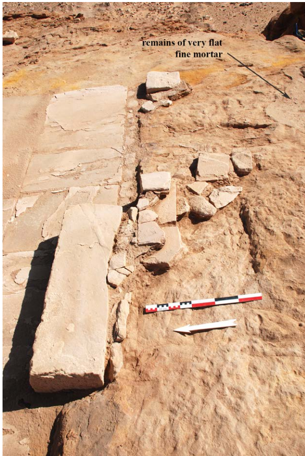
Fig. 11. Area immediately south of the platform. Levelling of the bedrock with stones, mortar and slabs.
