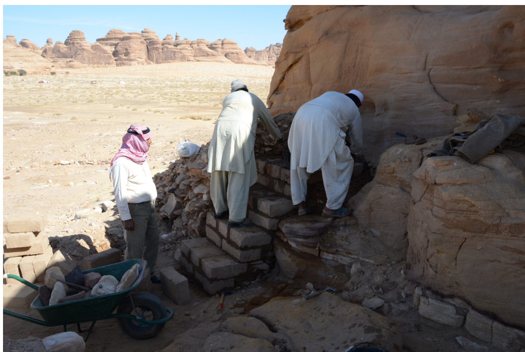
Fig. 24. Building of stairs giving access to the top of IGN 132.
