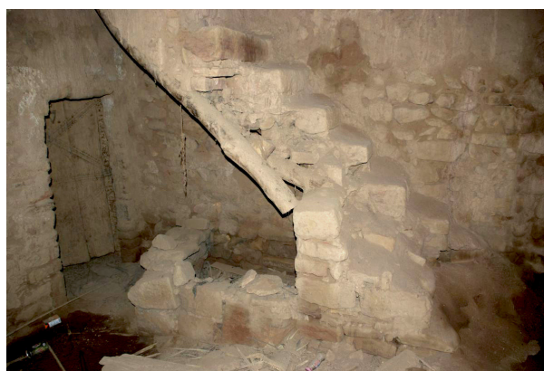
Fig. 9. Stairs in a house of ancient al-'Ulâ: note the storage compartment or trough under the stairs.
