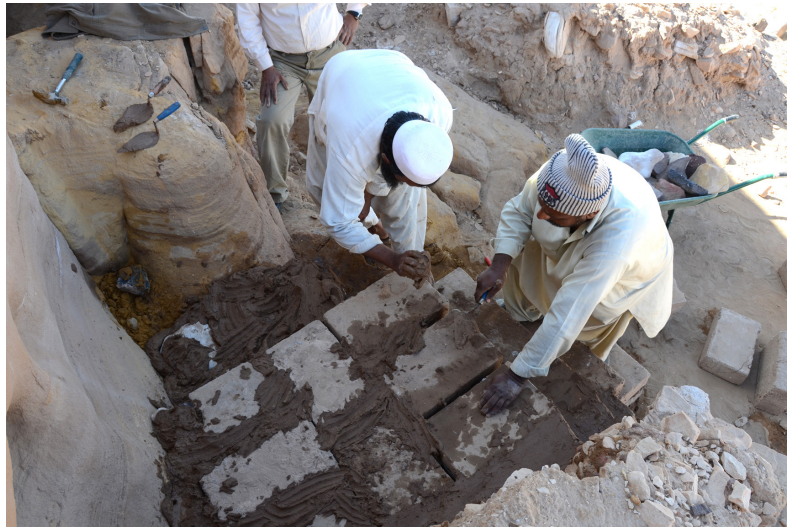
Fig. 1. Building of a staircase to give access to the top of IGN 132.
