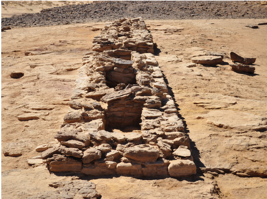
Fig. 22. Detailed view of wall locus 42003 after the excavation of the internal compartments, towards the south-west.
