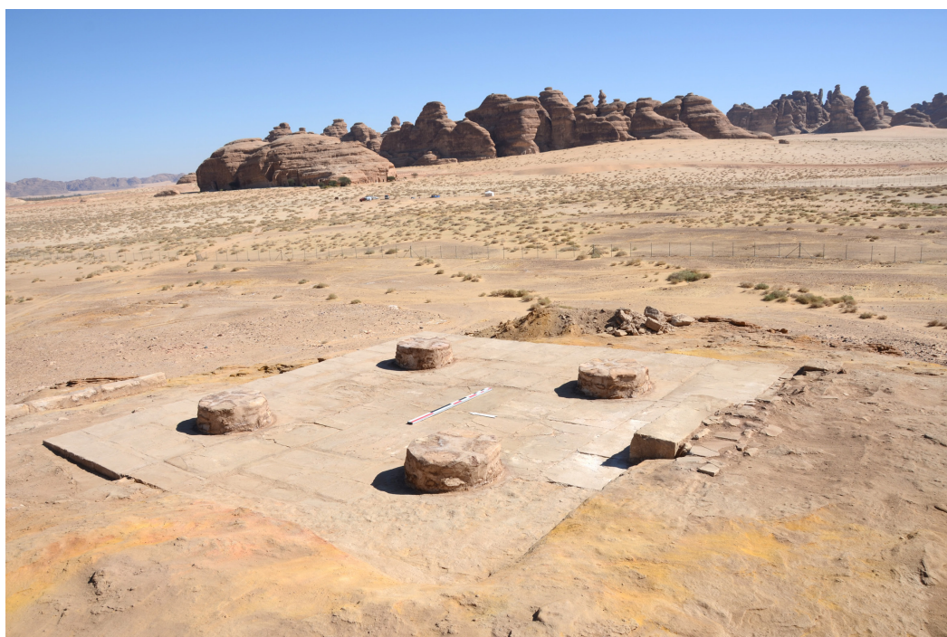
Fig. 25. Platform with tetrapylon after restoration at the end of the 2014 season.
