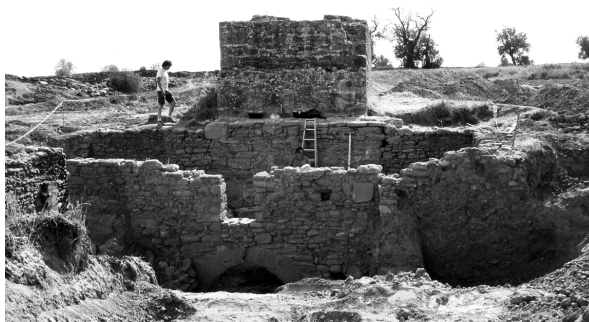
Fig. 4: The water mill of Palaiomylos
