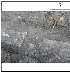
tranchée 8, mur M502
