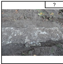
tranchée 8, mur M502
