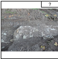
tranchée 8, mur M502
