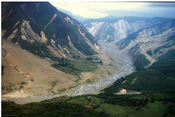
Figure 5: Effects of the earthquake and the flood of the river Paez - Tierradentro, Colombia. Source: http://enosaquiwilches.blogspot.com/2010/02/aprendamos-del-agua.html
