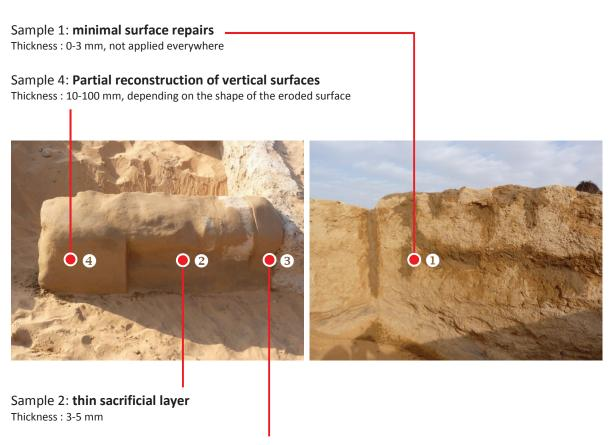
Sample 3: thick sacrificial layer, with or without reinforcement
