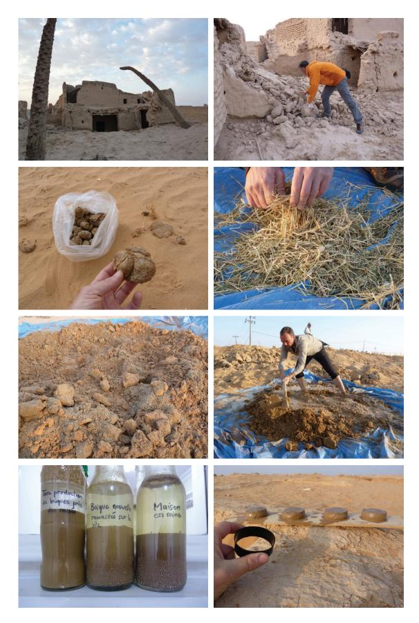
Photos illustrating the mortar preparation
