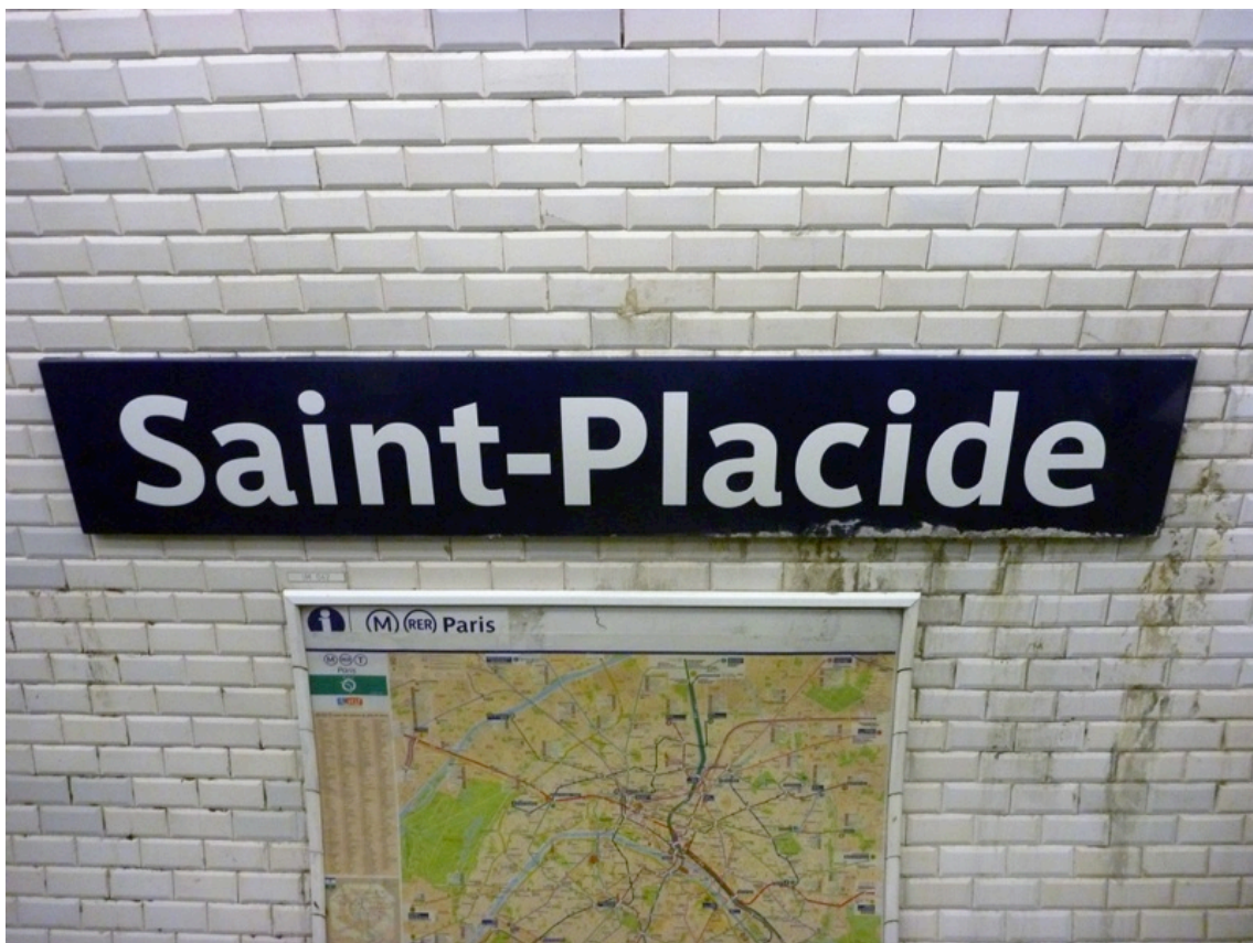
Figure 3. Mold on a signboard
