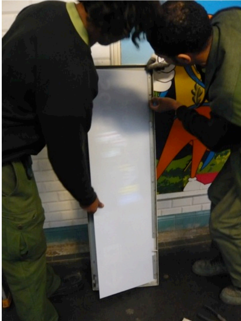
Figure 1. Disassembling a signboard
