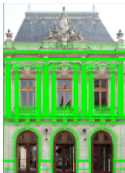
Figure 6: Using a set-upright picture for the 3D reconstruction. Here is a classical auditorium in Nancy (France).
