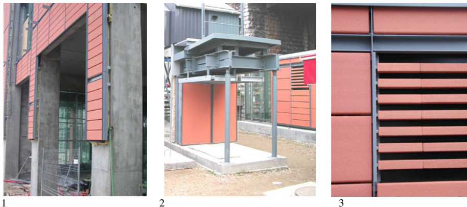
1 Building site of the Cité internationale in Lyon and experimental prototypes. Photo N° 3 : variations of the brick component.
