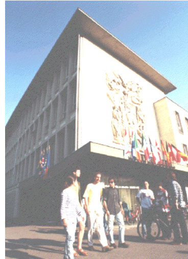
Figure. 4. Test building (ENSAIS)
