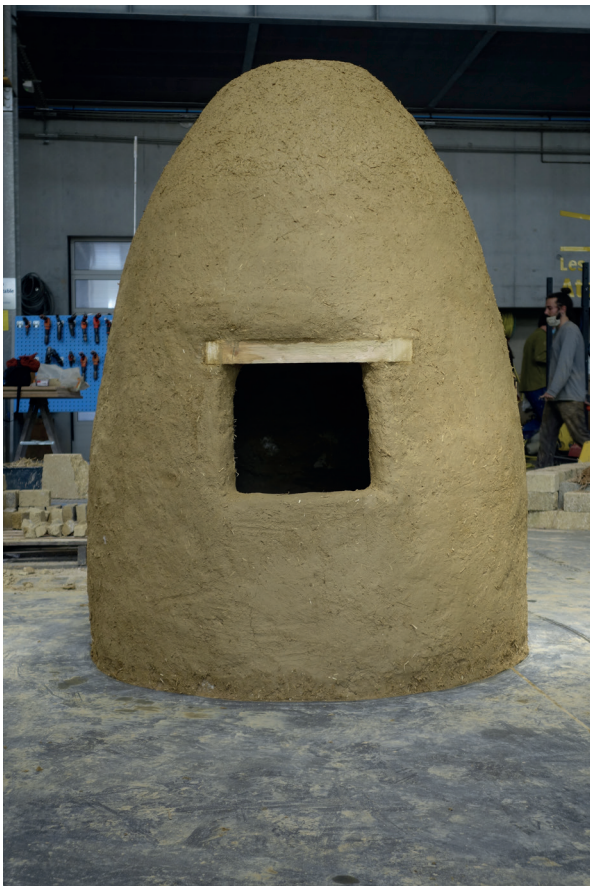
Figure 6. The first silo prototype at the end of the experimentation. © Adeline Bats.
