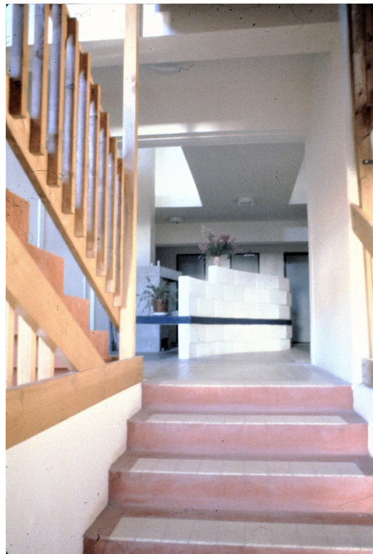
Figure 11. The common circulations, with a guardrail in the foreground designed and built by the inhabitants after the reception of the project, in replacement of a metal guardrail. In the background, the concrete bench decorated with plants with its chimney in front (archives architecturestudio).
