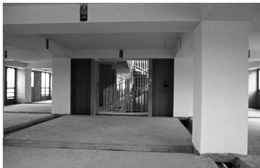
Figure 2. Les Marelles : Photograph of the raw plateau at the end of phase 1 before the interior layout chosen by the future inhabitants (DAF, CAPA, Archives Maurios).
