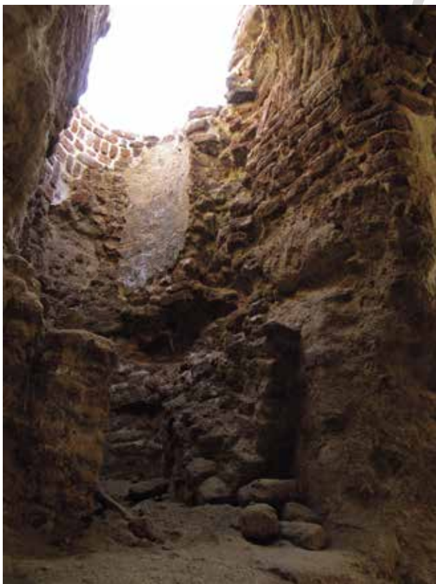
Fig. 11. Marea's double baths: central high-flame furnace mouth, under the boiler, from the subterranean corridor (Th. Fournet, 2005).
