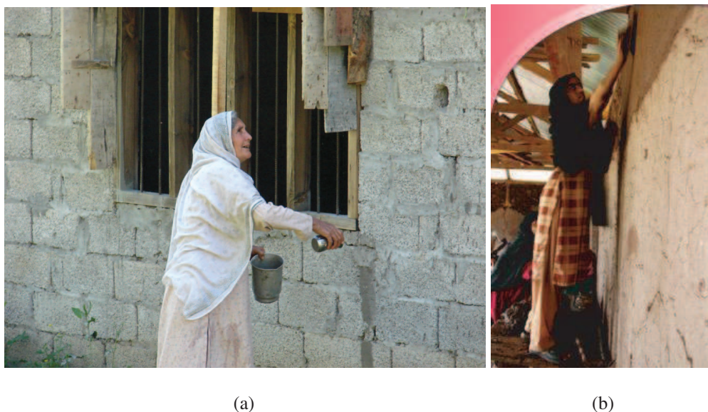
Figure 5.44 — Women also participated in reconstruction activities. (a) Source : ([Gallery, 2007]) ; (b) Source : ([UNHABITAT, 2007]) .
