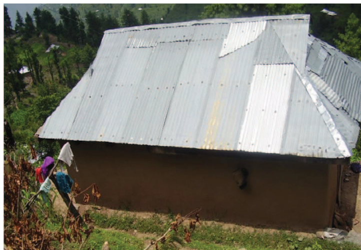
Figure 7.17 — Small pieces of CGI sheets are fixed through nails and bolts. Source : S. Abidi
