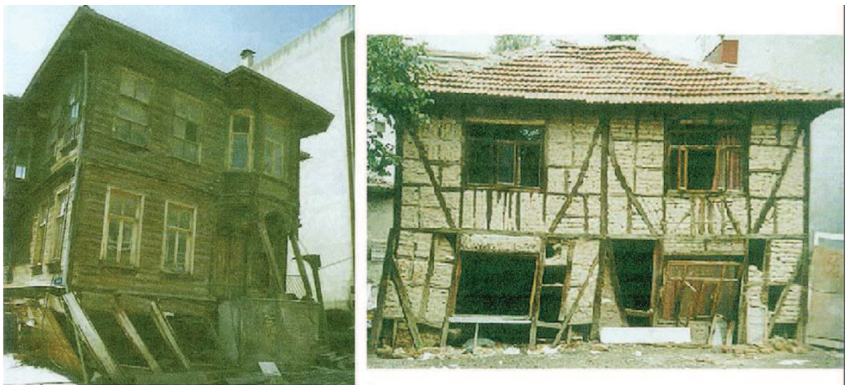
Figure 8.28 — Heavily damaged traditional wooden buildings due to soft storey. Left : Large laterally displaced traditional building ([Bayulke, 2004]) ; Right : Laterally displaced traditional building ([et al, 1999])
