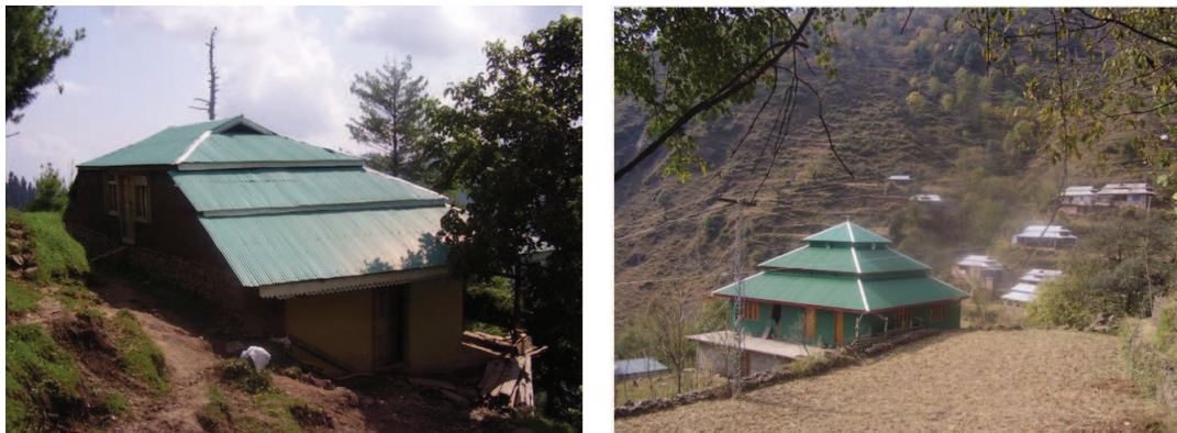
Figure 6.72 — Although negligible break in the roof is evident, the span of the roof has increased the height of attic. Source : S. Abidi
