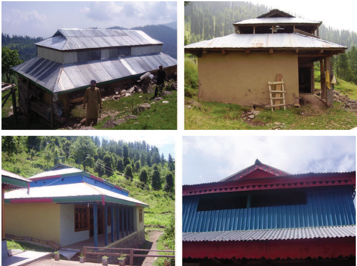
Figure 6.35 — A prominent break in the roof, Dutch Gable roof can be observed Above.
