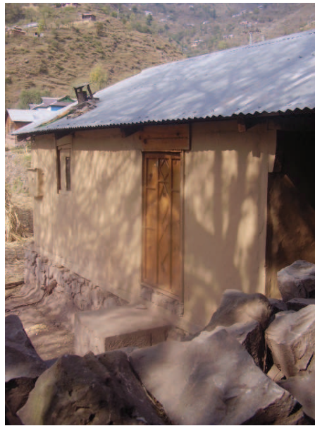
Figure 6.53 — Another single storey house in Muzaffarabad. Source : S. Abidi
