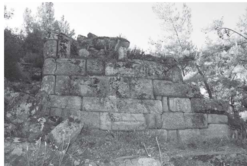
Fig. 51 : Parement sud de la Tour 4 (B. Vergnaud).
