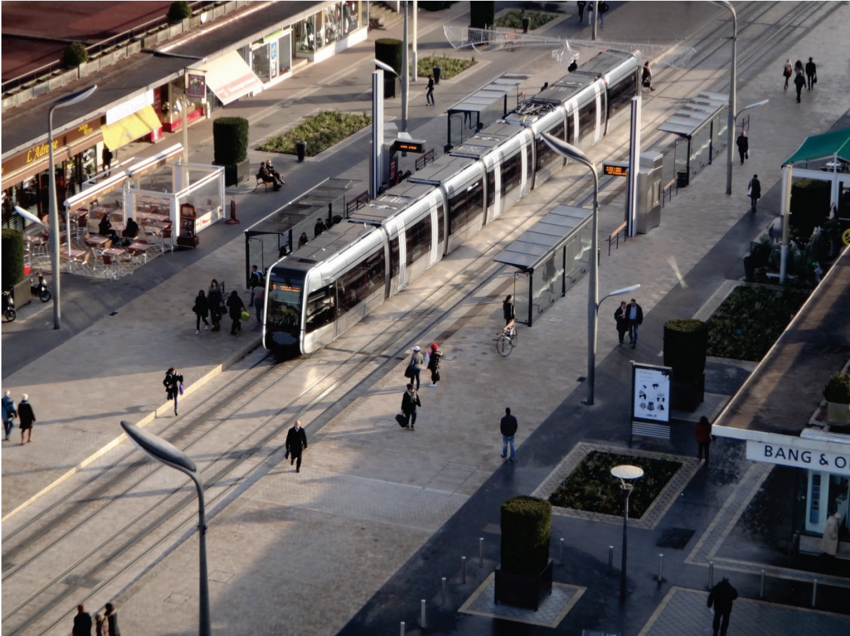
Station de tramway Anatole France (photo J.M. Beauvais)
