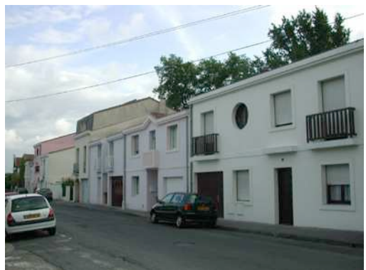
Figure 20 - Detached single-family housing development, Bordeaux, Mazières architectes, 1982. ©Ch. Callais
