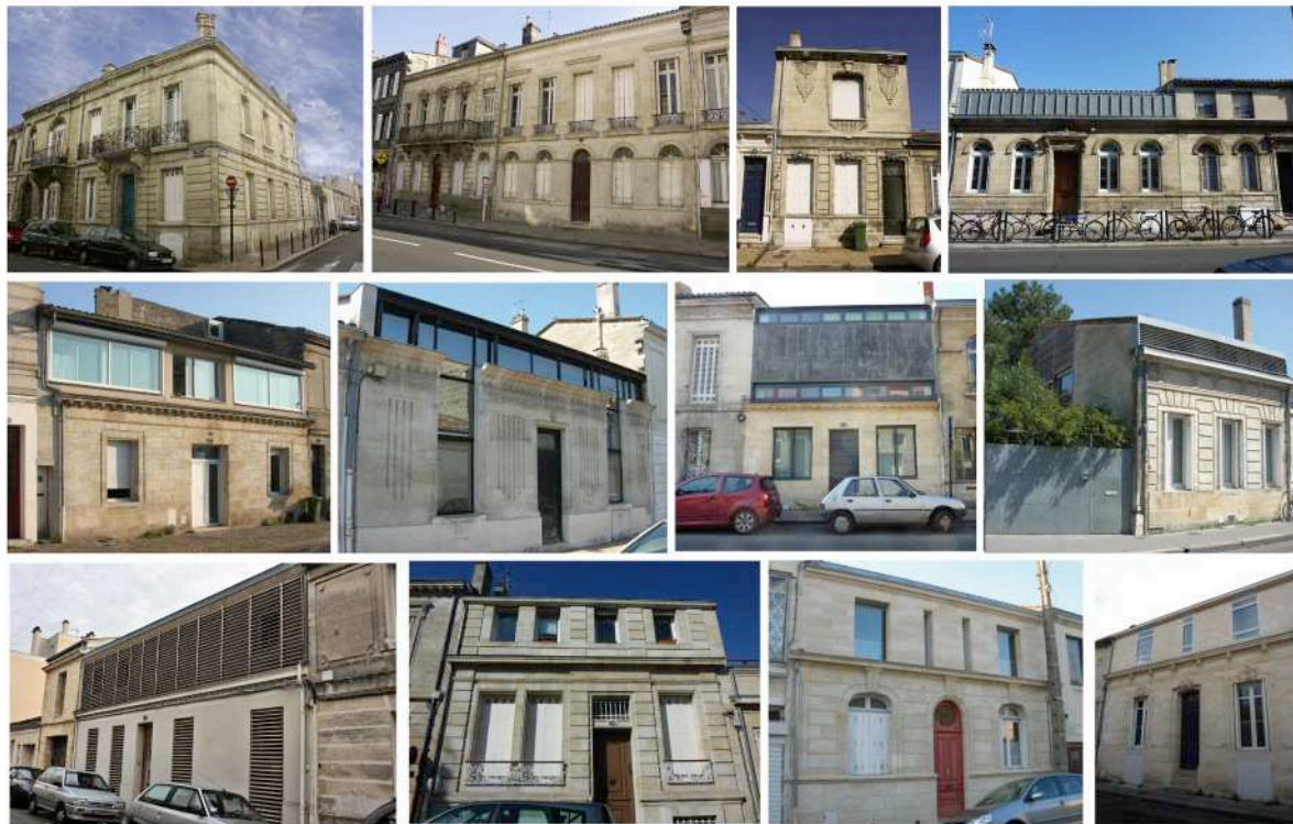
Figure 14 - House heightening by adding a floor: imperceptible in the 19 th and first 30 years of the 20 th century, diverse and posing aesthetic problems in the twentieth century. The “return of stone”; Today, stone is preferred and reintroduced as construction material. ©Ch. Callais and C. Pascual
