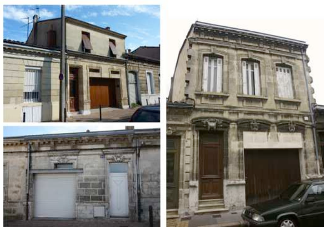
Figure 18 - Wall piercing for the construction of garage doors. ©Ch. Callais
