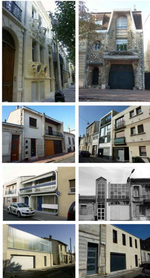
Figure 15 - Architectural renewal: adapting to the style of each period, examples from 1900 to present. ©Ch. Callais
