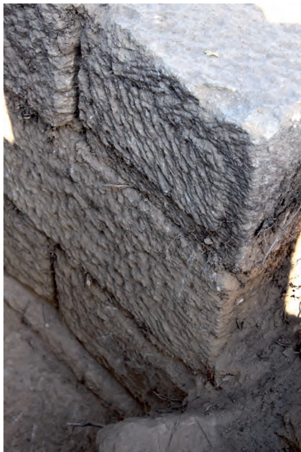
Fig. 14. View of the masonry of the east room. Note the carefully pointed surface and the drafted margin of the upper header.
