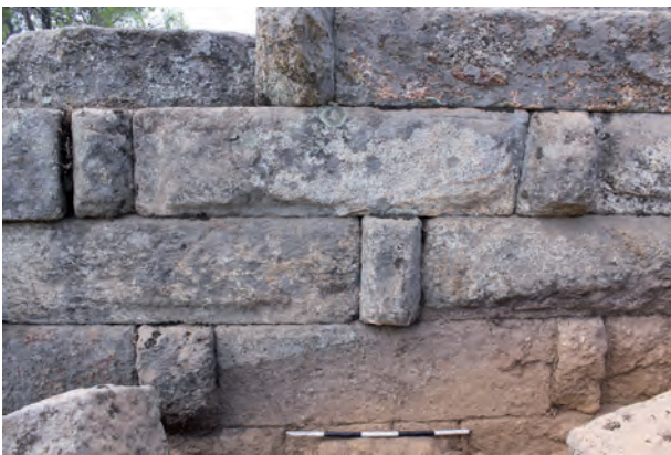
Fig. 6. Hekatomnid header-and-stretcher masonry of the central tower.
