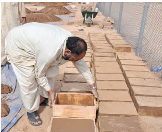
Fig. 13.16 Removal from the mould
