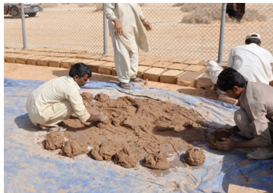
Fig. 13.13 Clods of earth prepared for the filling of the mould
