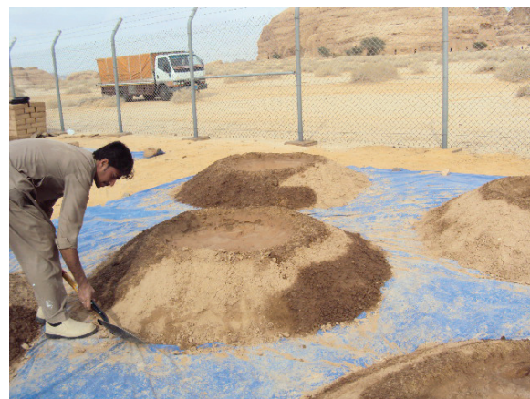
Fig. 13.6 Bringing the earth up on following morning
