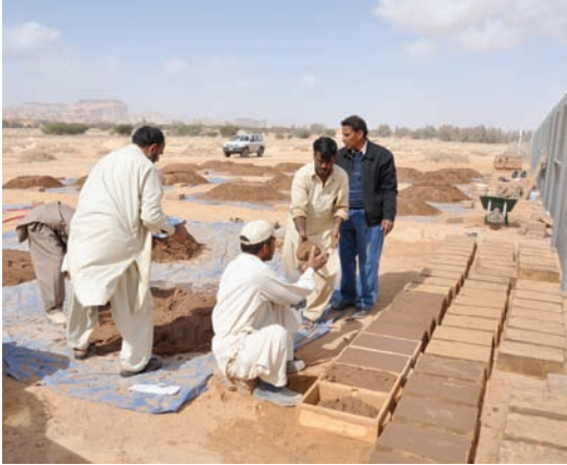
Fig. 13.14 Filling of the mould
