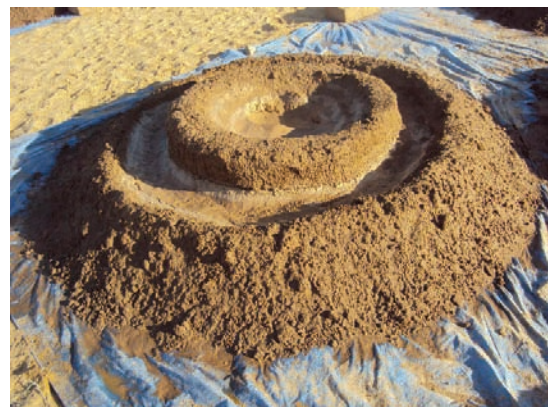
Fig. 13.7 Two-level crater to facilitate the wetting of the earth
