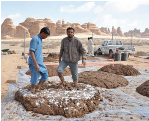
Fig. 13.10 Trampling the earth with the temper
