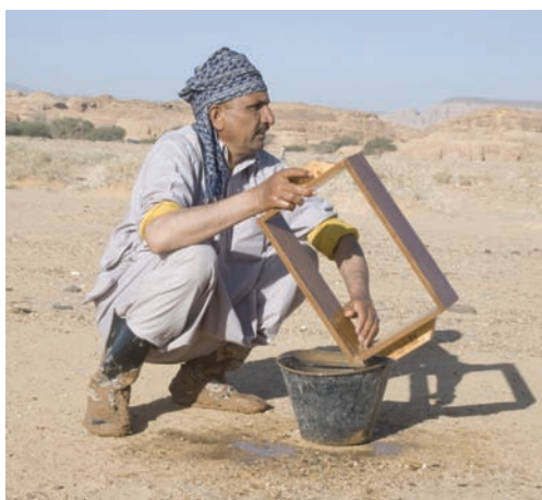
Fig. 13.12 Wetting the wooden mould
