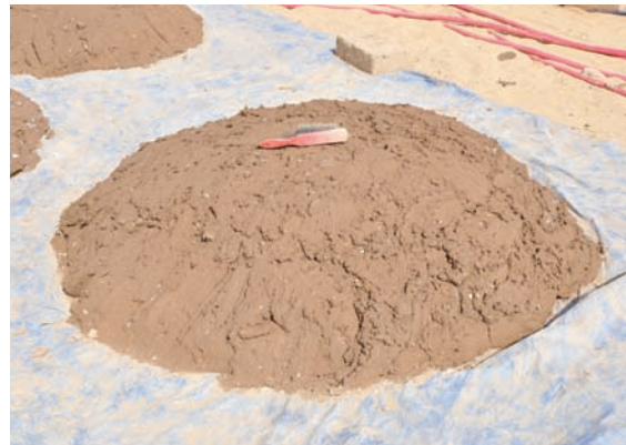
Fig. 13.11 Mound after mixing of earth with temper
