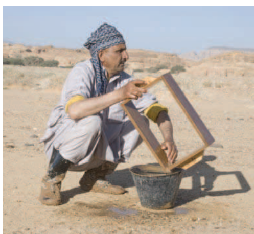
Fig. 13.12 Wetting the wooden mould
