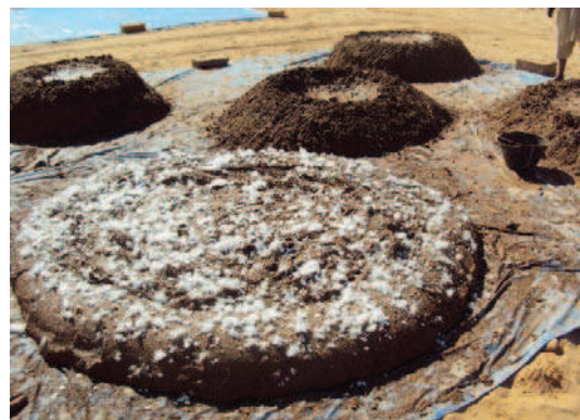
Fig. 13.9 Temper spread on top of trampled mound
