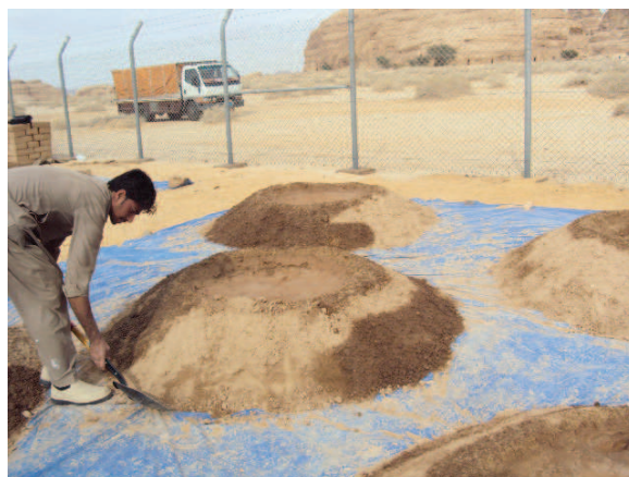
Fig. 13.6 Bringing the earth up on following morning
