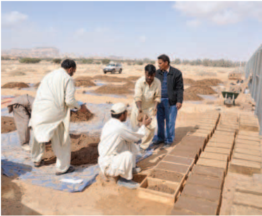
Fig. 13.14 Filling of the mould
