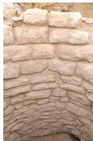
Fig. 46 The masonry of the well on the western side. Note the size of the ashlar, which are much larger at the top than at the bottom
