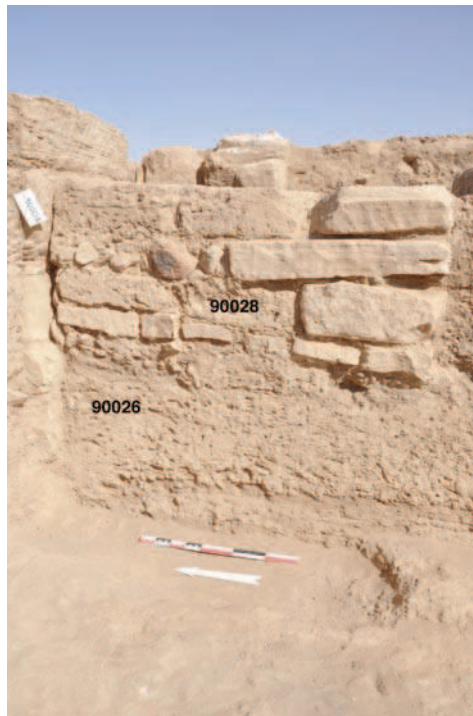
Fig. 28 Trench A. Wall 90028, from the south-west. In the extreme left is the corner section of wall 90030
