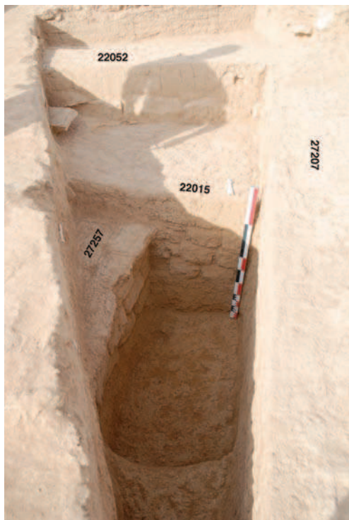
Fig. 16 Intersection of walls 27257 and 22015, viewed from the south
