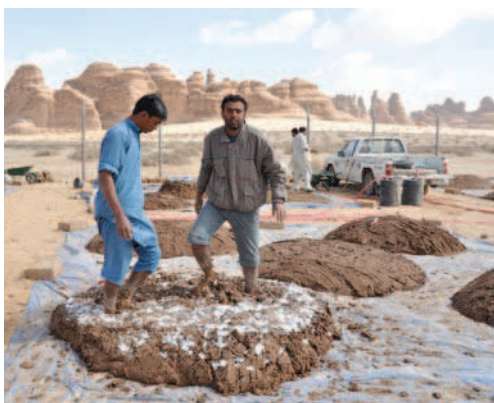
Fig. 13.10 Trampling the earth with the temper
