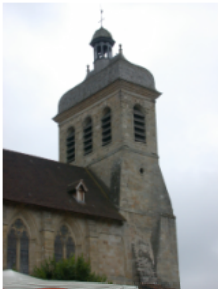
Figure 3: Outside view of the abbey church.
