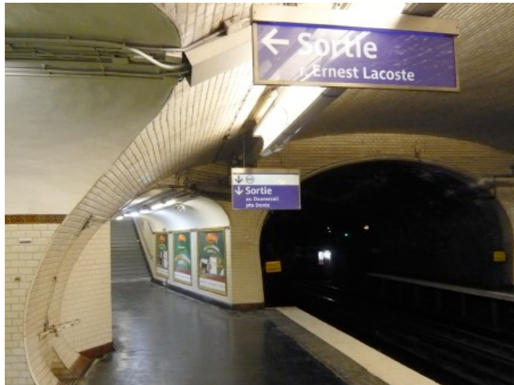
Photo 3. Exit boards to be replaced to include the museum name
