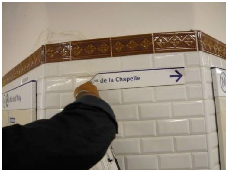
Photo 14. Removing a provisory board
