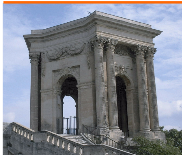
Figure 5. The Water Tower
