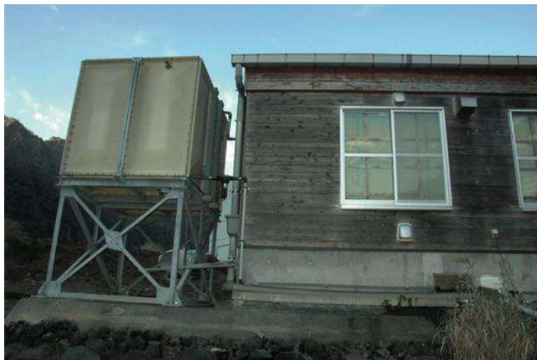
PHOTO 6 10-ton Raw Seawater Tank with a Filter. A seawater pipe extends into the saltworks through the filter from the seawater tank (left) and saltworks building (right) from the bottom right of the tank.
